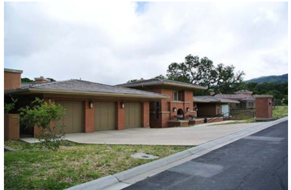
Nearby House on Santella Court
